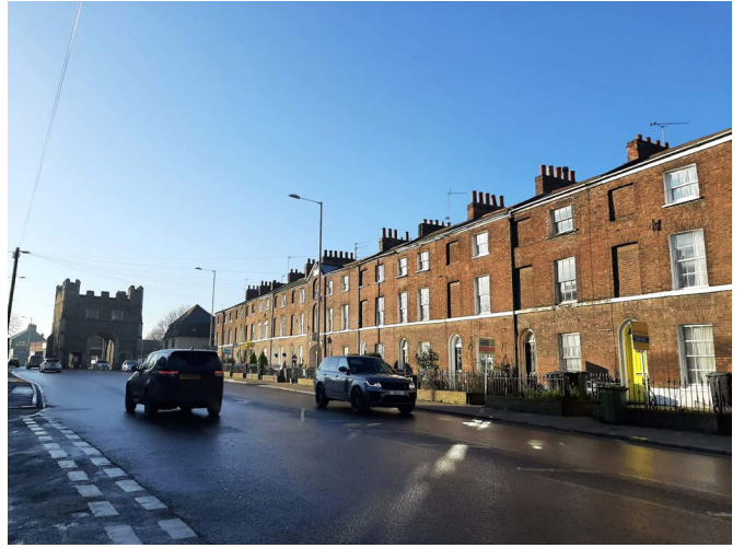
Grade II Listed Buckingham Terrace, London Road
