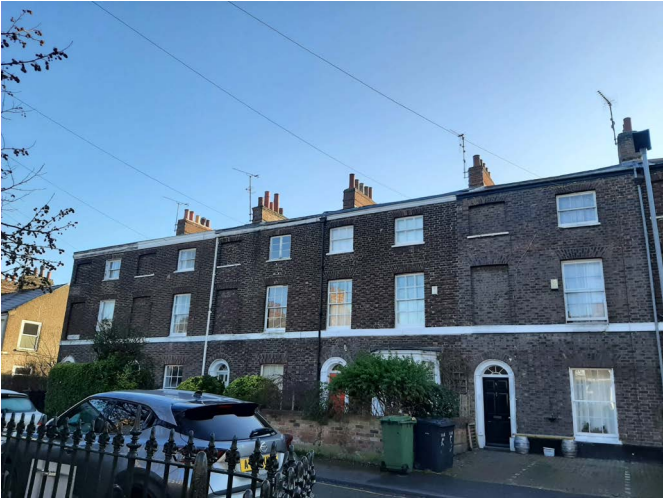
Grade II Listed 1-11 Guanock Place, London Road
