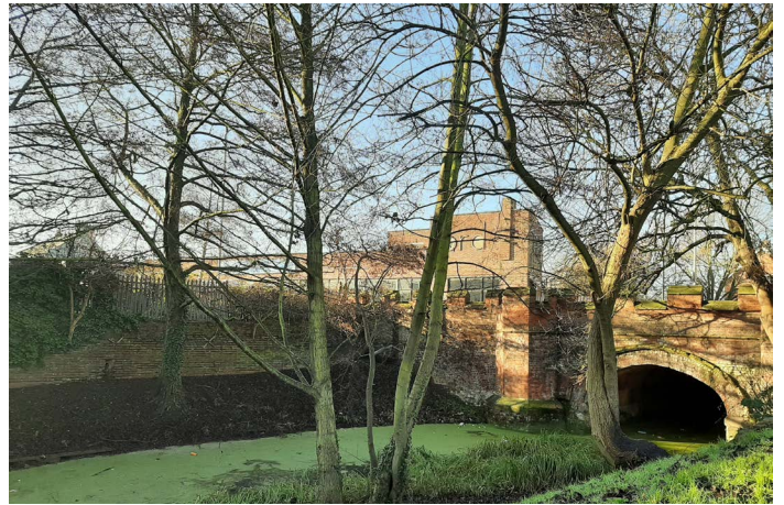
Middleton Stop Drain, Southgates Park
