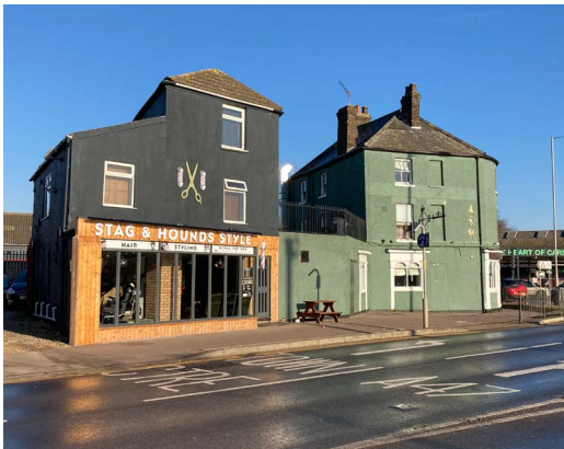
Former Prince of Wales Public House
